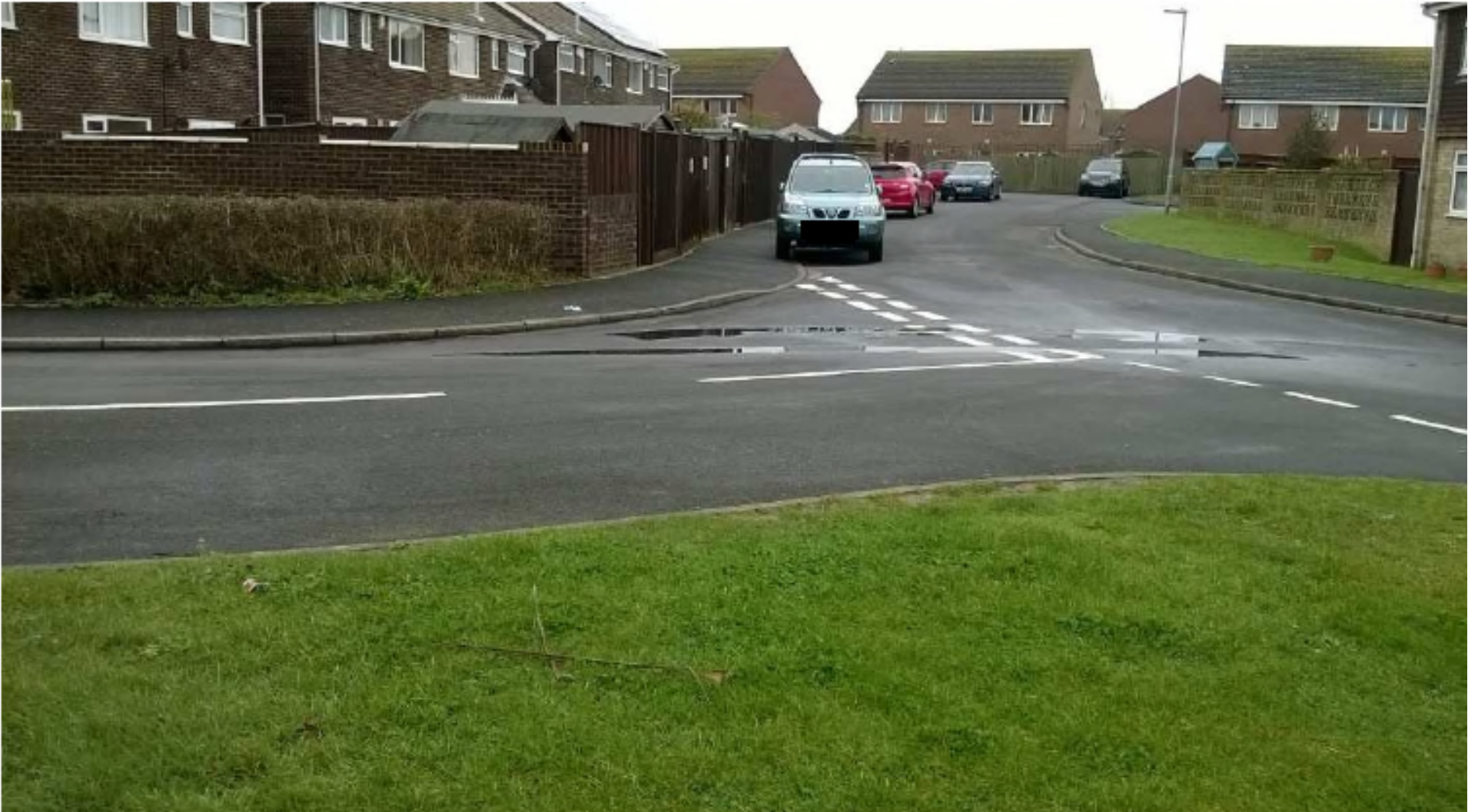
View 3 – Looking eastwards towards the Aylesbury Avenue junction
